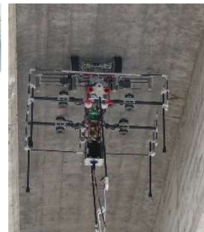
(h) Drone with wheel for visual observation and hammering tests
