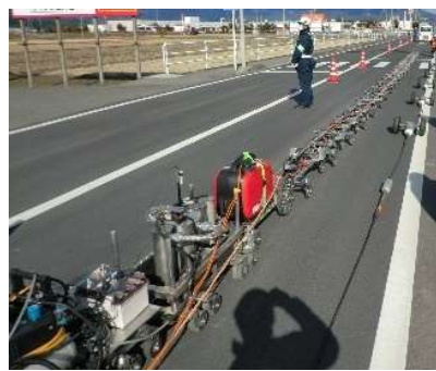
(c) Pavement inspection system using surface-wave and electric-resistivity
