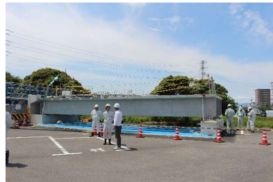
(a) Prestressed concrete bridge
