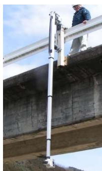
(b) Robotic camera indicating crack scale for bridge inspection
