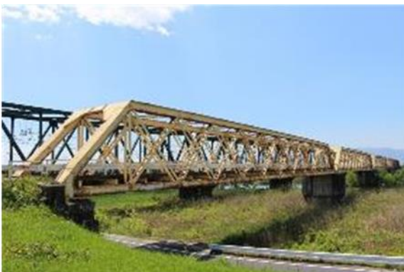
(a) A view of the entire bridge.
