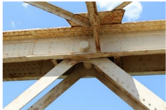
Figure 7. Panel point of truss bridge.
