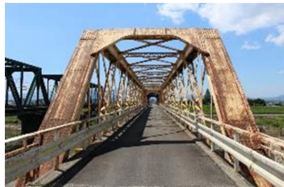
(b) Road Surface.
